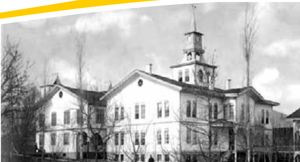
Merzifon Main Building
