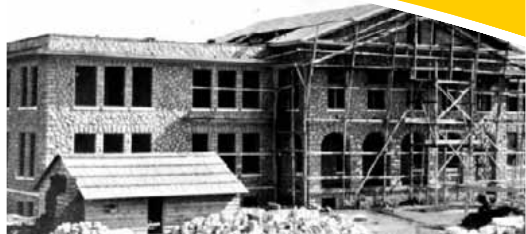
Construction of Macedonia Hall, 1930-1934
